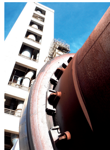
Rotary kiln 3 and preheater tower at the cement plant LEUBE.
